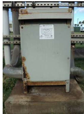
Corroded Transformer
