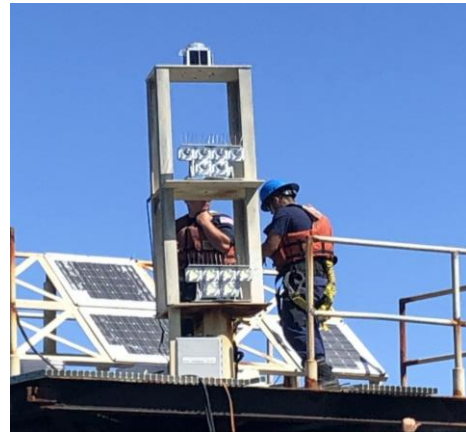
Coast Guard crew members from Aids to Navigation Team Mobile and Coast Guard Cutter Saginaw repair Mobile Alfa Range Front Light, September 28, 2020, following Hurricane Sally. (Coast Guard photo)
