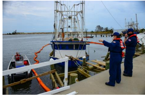
In the aftermath of Hurricane Sally, Petty Officers from Coast Guard Sector Mobile, assess damage and oversees contractors tasked with booming off and cleaning up oil and fuel leaks in the water near downtown Pensacola, FL, September 19, 2020. (Coast Guard photo)
