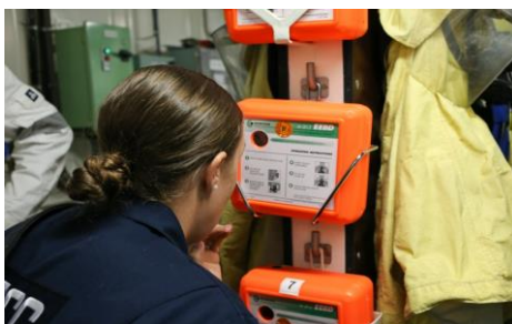
A Coast Guard Petty Officer examines an emergency escape breathing device (EEBD), during an inspection aboard a gas carrier vessel near Freeport, TX, December 13, 2019. (Coast Guard photo)
