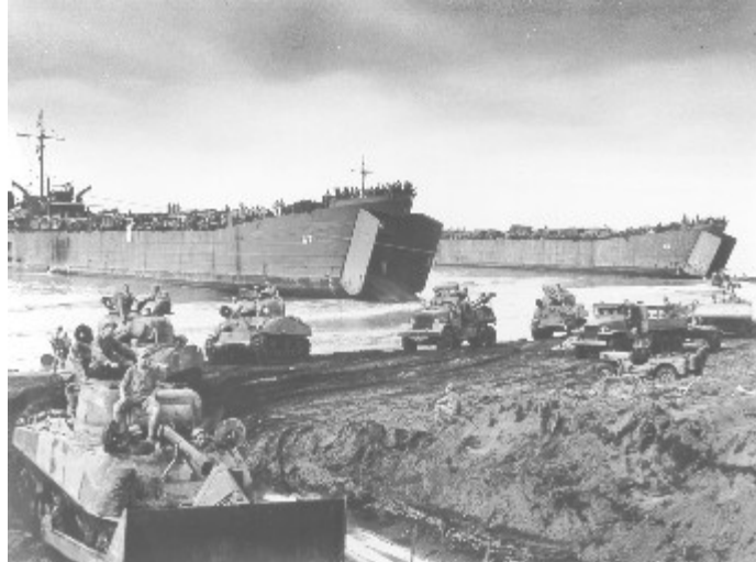
"CG brings tanks. . ."; no date (July, 1944?); Photo No. 2642; photographer unknown.
