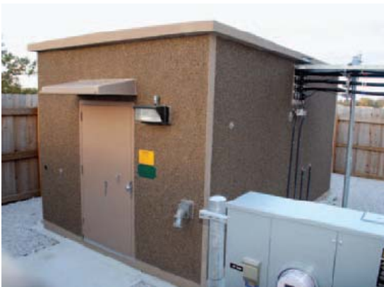
Fig. 2-4 Example of a typical communication shelter.
